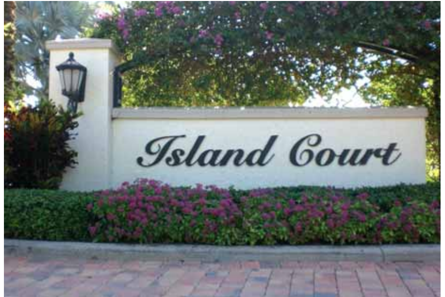
5-by-10-ft. double-face concrete sign with an HDU cap and copy. Column at left is 2-by-7-ft. and is built from HDU and overlaid plywood fastened to the existing concrete structure
