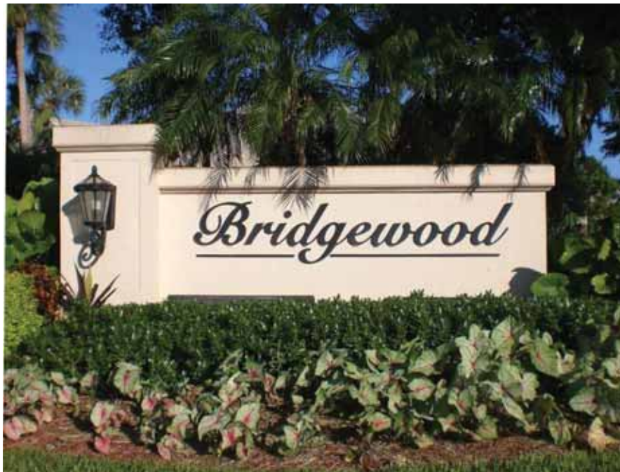
5-by-13-ft. concrete structure with HDU cap and copy. The column at left is 2-by-6-ft.
