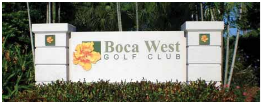
Sign face is 6-by-11-ft. and made of HDU laminated to overlaid plywood. The copy is cut from aluminum.
